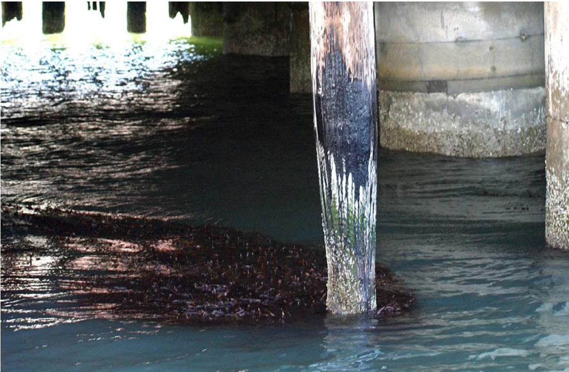
Figure 3-1. Visible creosote slick detected during field mapping in San Francisco Bay. (project team photograph)
