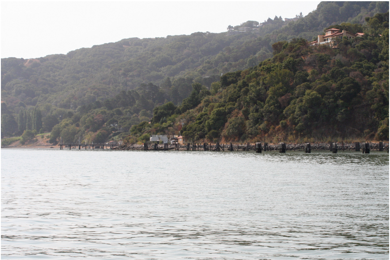
Figure 6. Abandoned bulkhead, 2008. (Courtesy of NOAA)
