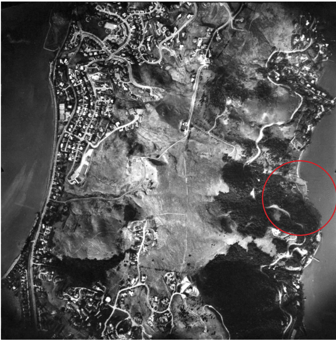
Figure 5. El Campo, 1969. The marina was abandoned sometime between March 1967 and August 1968. Dividers between boat docks have been dismantled and very little remains of the site even in the late 1960s. Gangways can still be seen connecting the filled land to the marina. (Brady 1969, courtesy of Marin History Museum)
