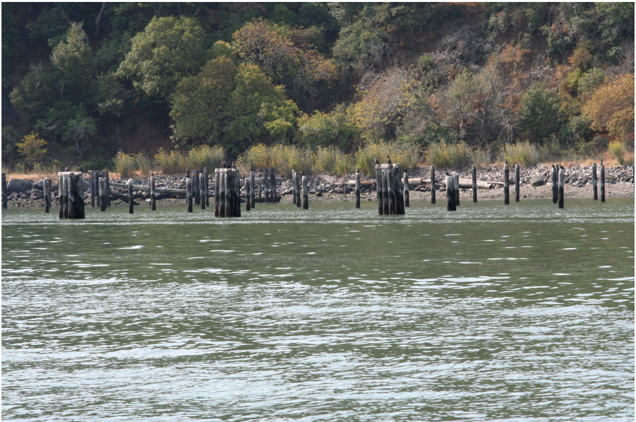
Figure 7. Abandoned bulkhead, 2008. (Courtesy of NOAA)
