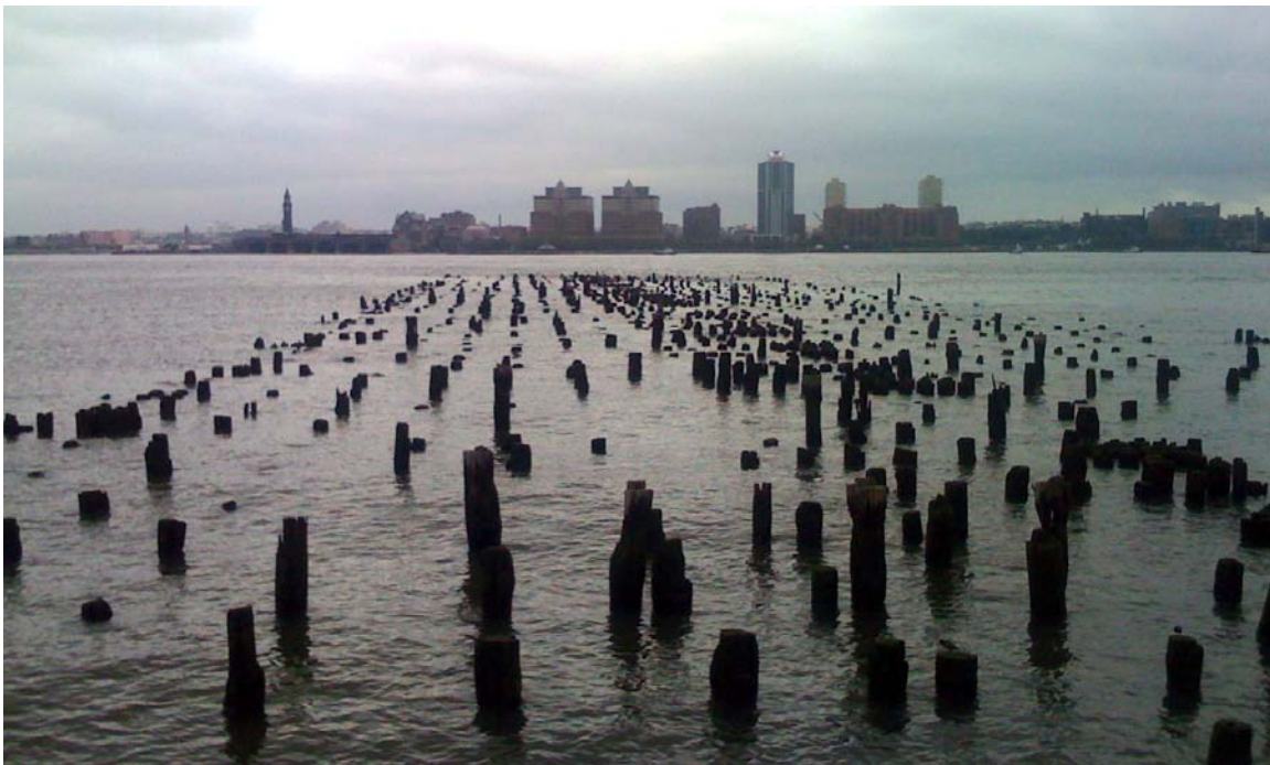
Figure 1-5. The Hudson River Park Trust removed decking but is committed to preservation of pilings as habitat for invertebrate and fish species. (project team photograph)
