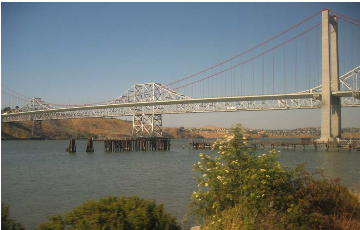
Figure 7-1. Old pilings may be hazards to navigation. (project team photographs)
