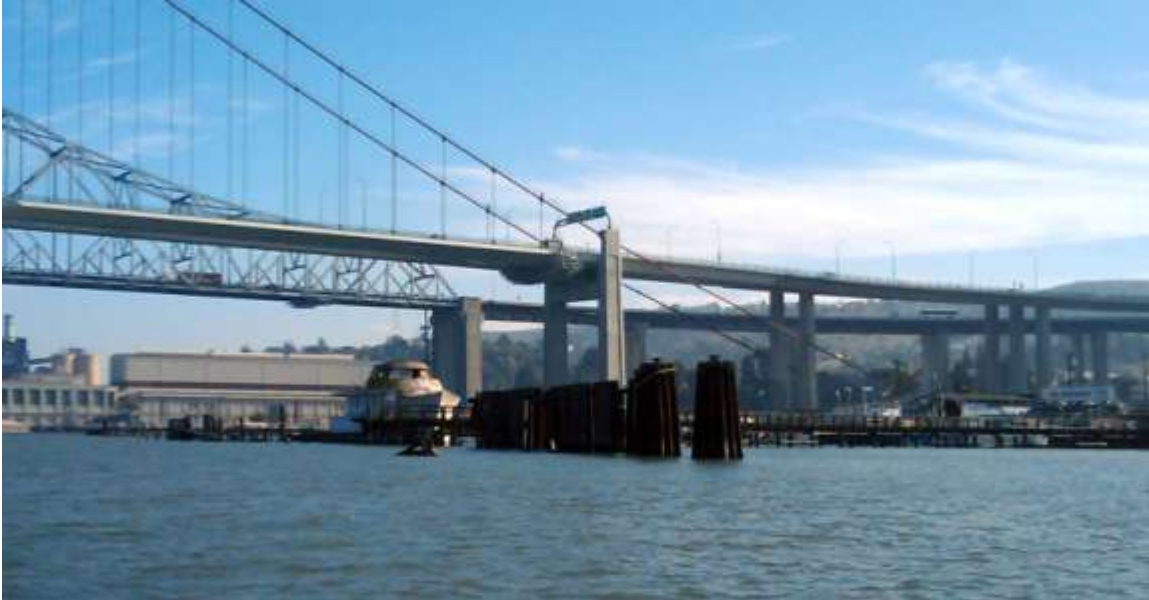
Figure 7 - Photo Taken beneath the south side of the Carquinez Bridge during QA/QC field work on December 11, 2008.
