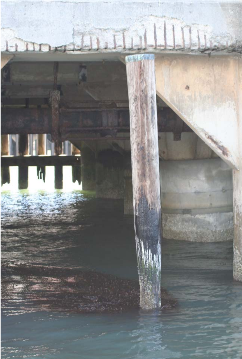
Figure 1. Creosote leaching from pier piling in San Francisco Bay as observed by NOAA survey 2008 (Photo credit: William Winner).
